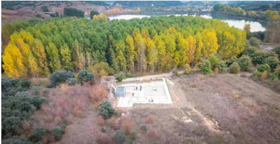
Fig.10. Aerial image of the intervention in the Domus Romana de Pedreiras de Lago, in Lago de Carucedo (Las Médulas, León) (Photo by LAB/PAP, 2019).
