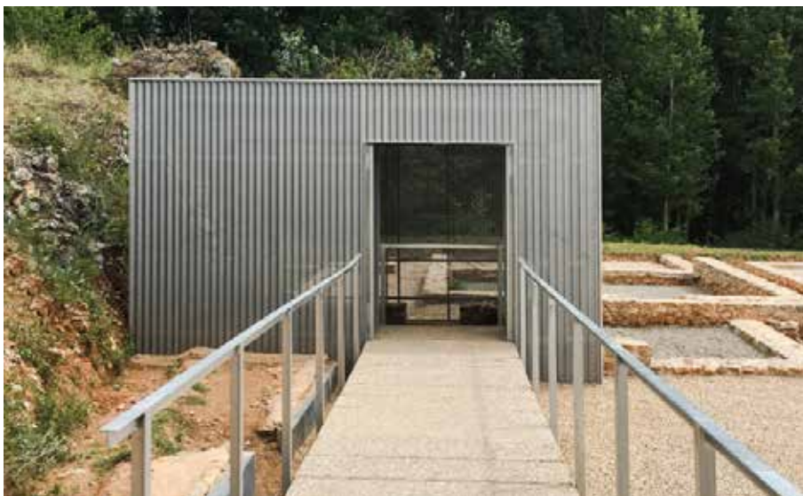
Fig. 12. Access walkway to the pavilion of the Domus Romana de Pedreiras de Lago, in Lago de Carucedo (Las Médulas, León) (Photo by LAB/PAP, 2018).
